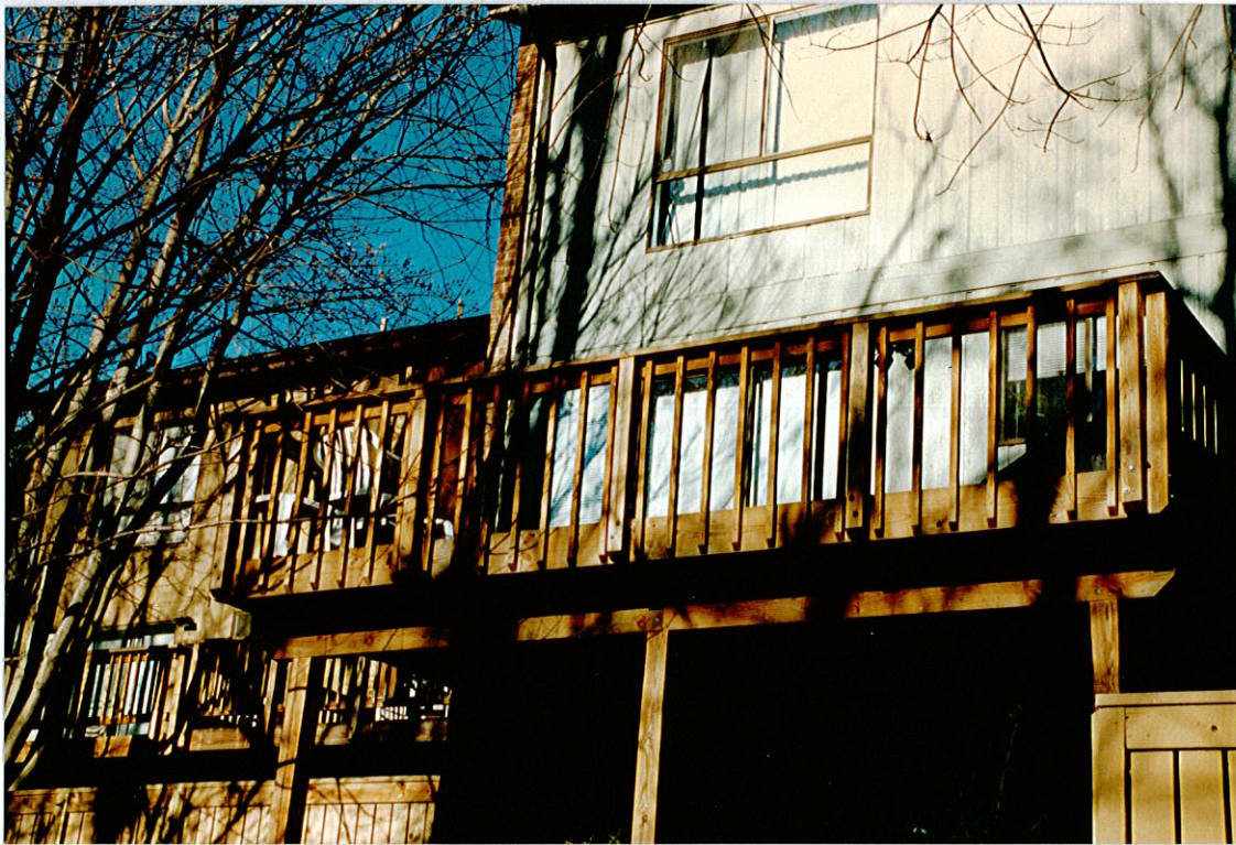
DECK, REAR (Close-up) (see specifications on next page)
